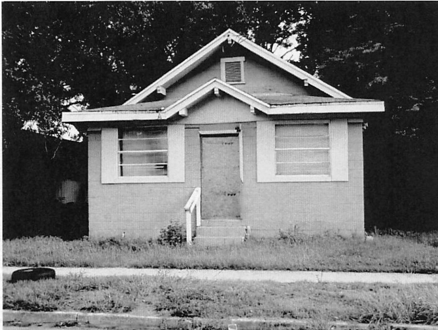
Adjacent residential structure
